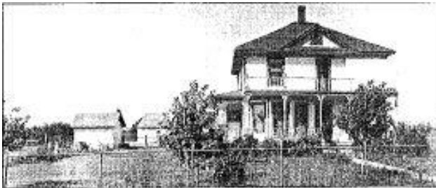
Home of Julie & George E. Wilson. Located north of 15th and Dalton, circa 1920. He had land to the base of Canfield Mountain and was an officer in the Fruit Growers Association. The house was built about 1915 to 1918 using all clear lumber. DG-1-15
