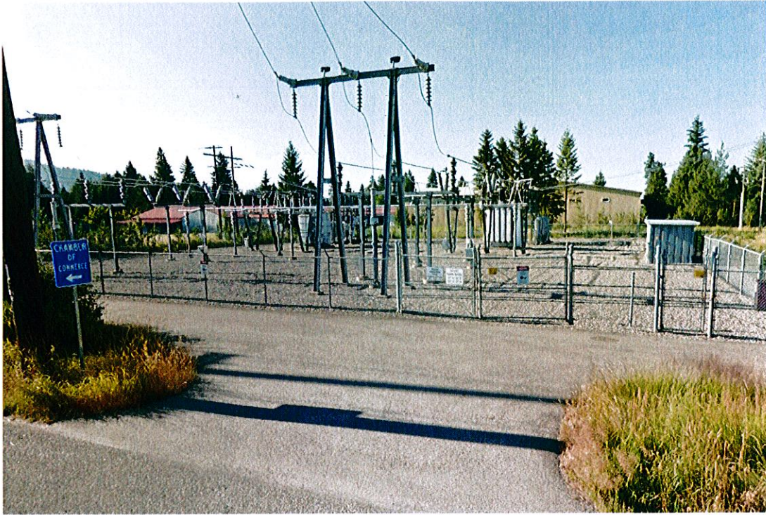
June 2019: 6-ft high chain-link fence with 3-strands of barbed wire
