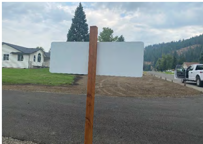
NO BRACE ANGLES / INCORRECT POST SIZE
