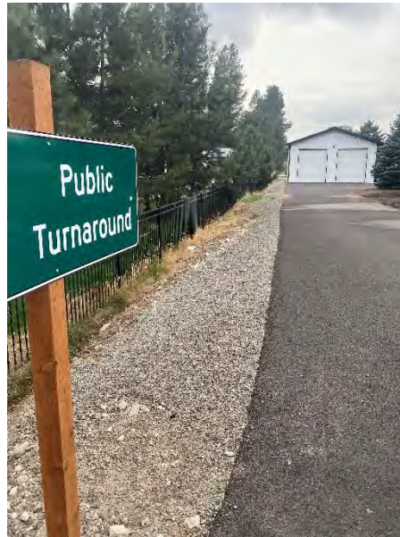
INCORRECT SIGN HEIGHT / MISSING NO PARKING SIGN
