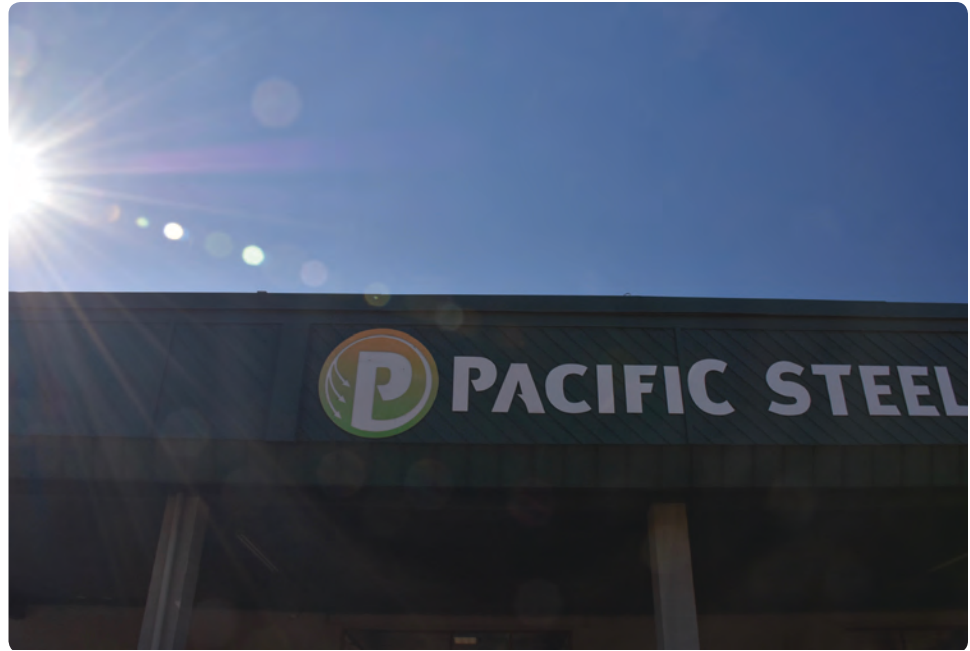
Figure 1.09 – Some of the buildings in the subarea are well maintained, with facades and sites consistent with a prosperous business environment. Others, however, show their age and lack of care, resulting in an uneven appearance along the corridor. (Source: SCJ Alliance.)
