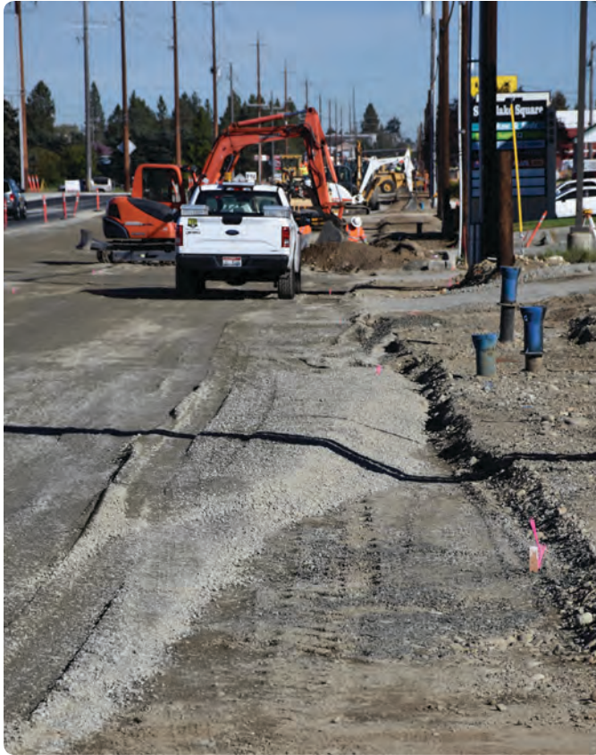
Figure 1.03 – Government Way improvements underway during this plan's preparation will widen the roadway and install curbs and sidewalks along the road's edge. (Source: SCJ Alliance.)
